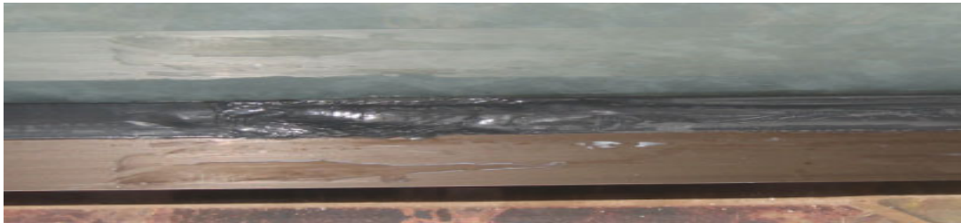
Typical Wet Glaze Installation Installed by Professional Caulker
